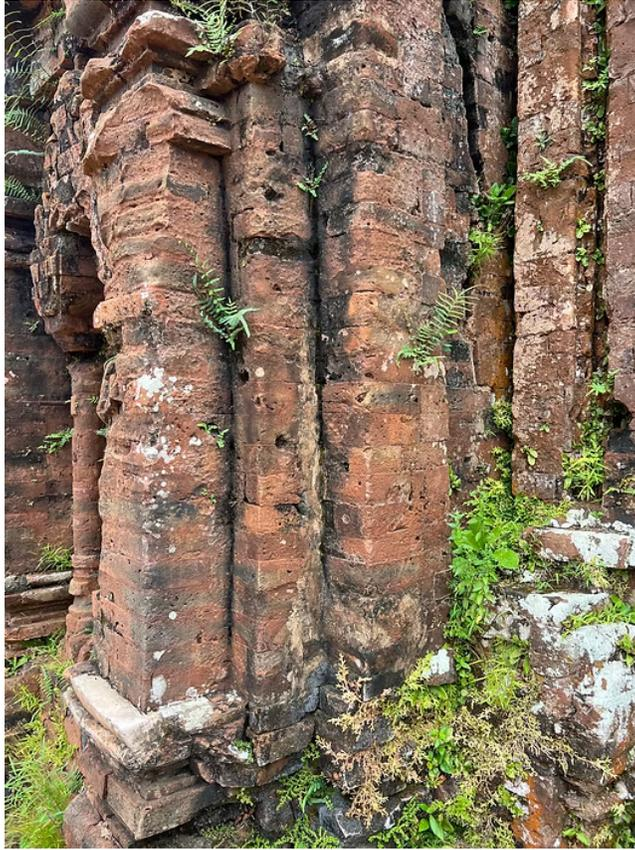
Done with zero mortar. Just brick on brick,
